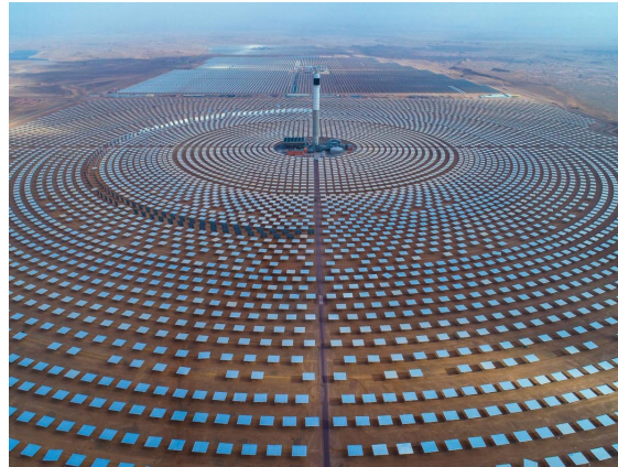
NOOR COMPLEX POWER PLANT (MOROCCO)
